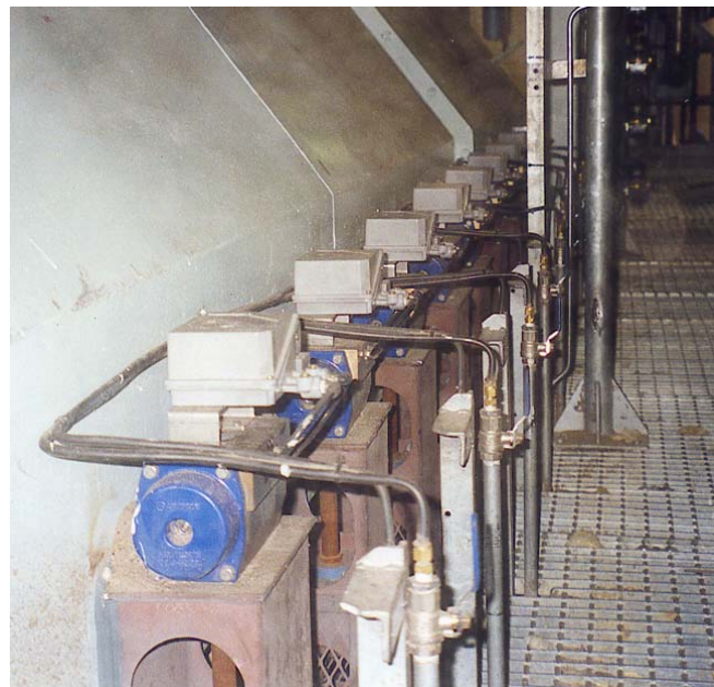
Fig. 7 : View of TES Auto-controlled Zoning Damper Operating Gear
